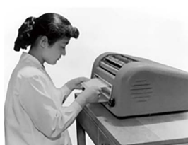
The Ricopy 101, Japan's first desktop diazo-wet copier to integrate exposure and development
