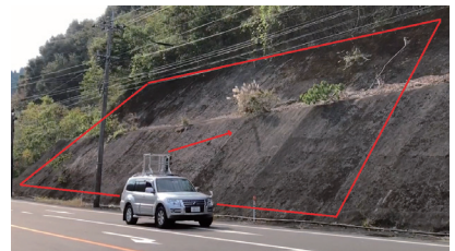
Image of slope surface
