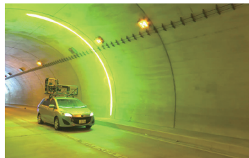
View of tunnel interior
