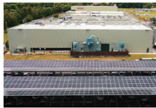
Private power generating equipment at a RE100 certified British plant
