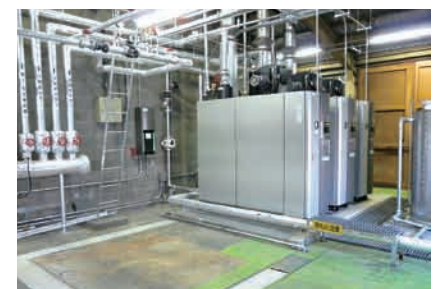
Natural gas boiler that takes up 60% less space than the previous boiler
