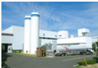
Natural gas supply by tanker trucks
