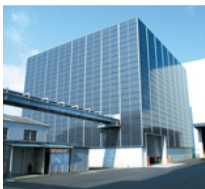
Waste water treatment equipment with solar panels on the exterior
