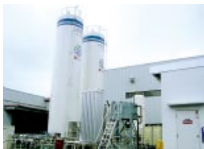
Exterior of the cogeneration system: Liquefied natural gas tank (left) and gas engine power generator building (right)
