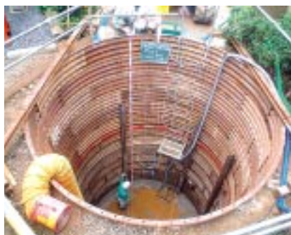
Removing polluted soil (at Ricoh Ohmori Office)
