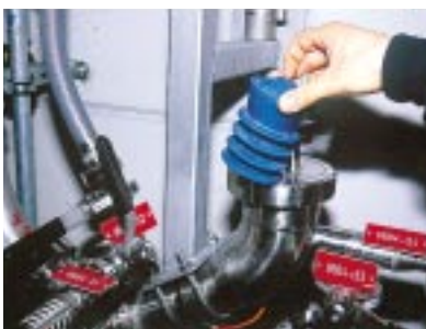
Cleaning the pipes pneumatically by putting balls inside the pipes
