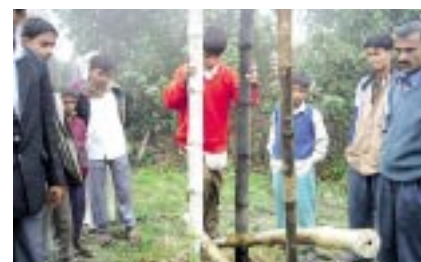
Installation of a treadle pump
