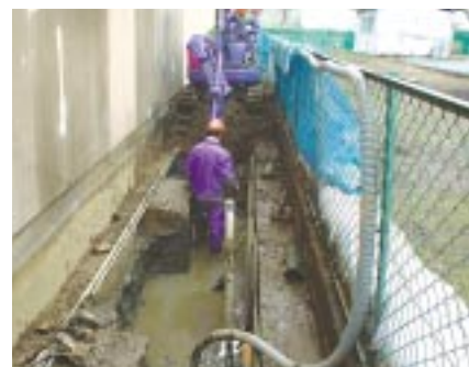
Soil improvement work at borrowed premises
