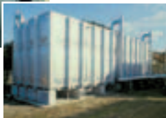
Ice thermal storage tank
