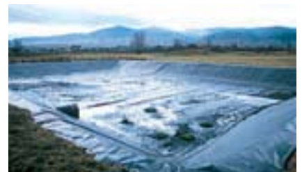
Water pool for fire fighting at Ricoh Industrie France
