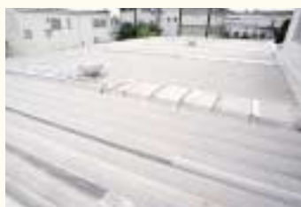
Roof painted with adiabatic paint
