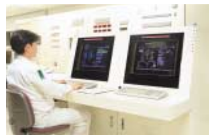
Safety control room at Ricoh Yashiro. This room monitors detection devices throughout a plant. In an emergency, appropriate instructions are immediately given from the control room, accompanied by an alarm and a warning on monitors.
