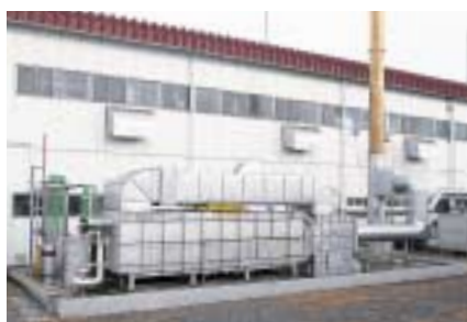
Direct solvent gas burner
