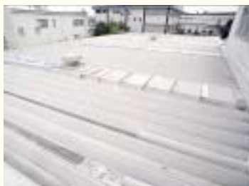
Roof painted with adiabatic paint
