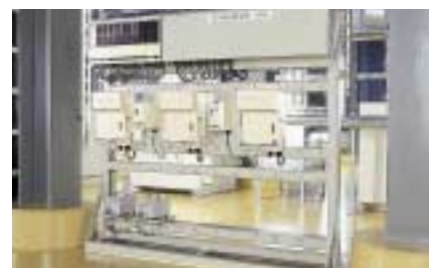
Gas sensor unit at Ricoh Yashiro. This device is designed to detect gas leakage, with relevant data monitored constantly in a control room.
