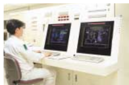
Safety control room at Ricoh Yashiro. This room monitors detection devices throughout a plant. In an emergency, appropriate instructions are immediately given from the control room, accompanied by an alarm and a warning on monitors.
