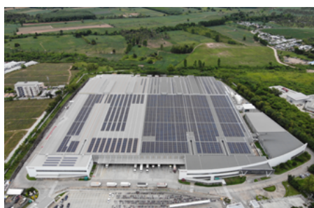
Roof of Ricoh Manufacturing (Thailand) Ltd. plant
