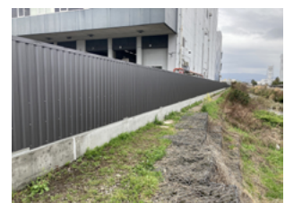
Installation example of flood wall at Ricoh Numazu Plant
