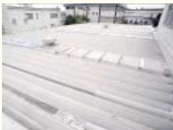
Roof painted with adiabatic paint
