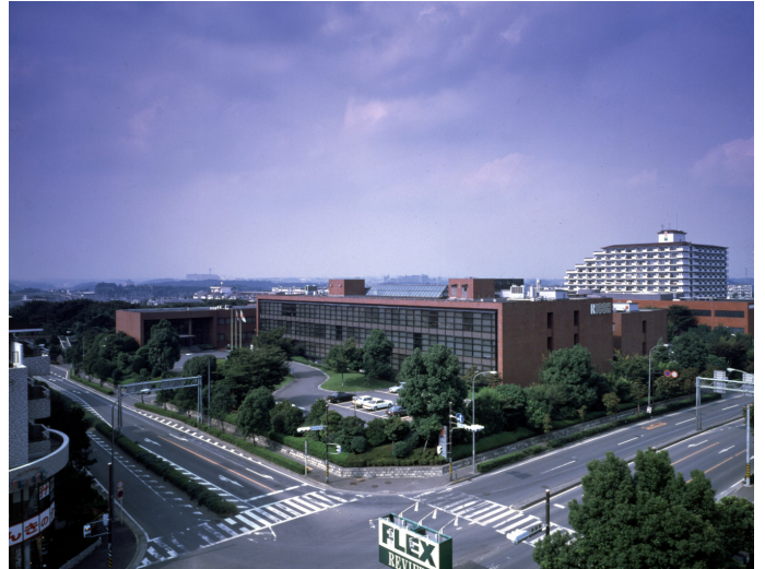
Ricoh Research and Development Center is located in an area of lush greenery
