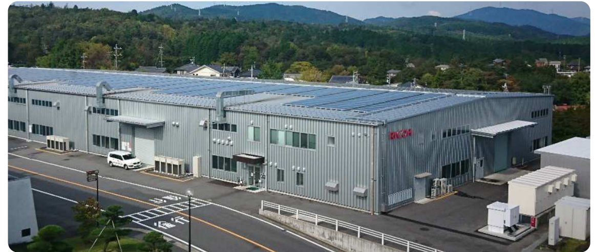
Ricoh Elemex Ena Plant Rooftop
