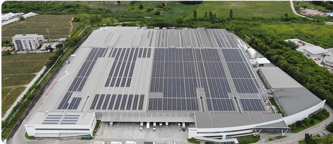
Rooftop of Ricoh Manufacturing (Thailand)
