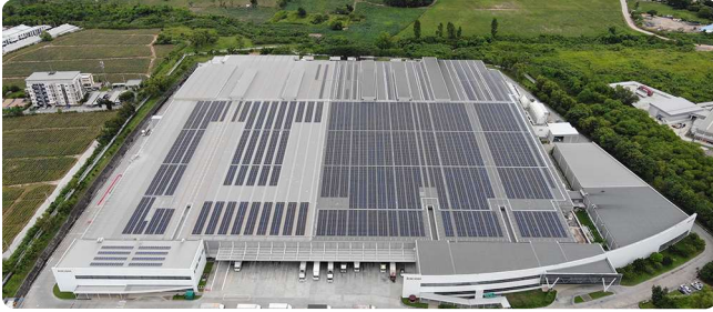
Rooftop of Ricoh Manufacturing (Thailand)
