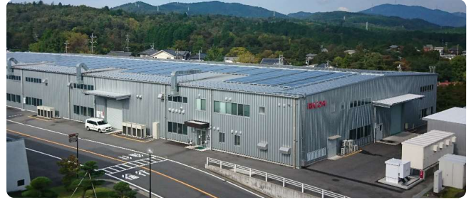
Ricoh Elemex Ena Plant Rooftop
