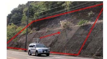
Roadside slope monitoring system
